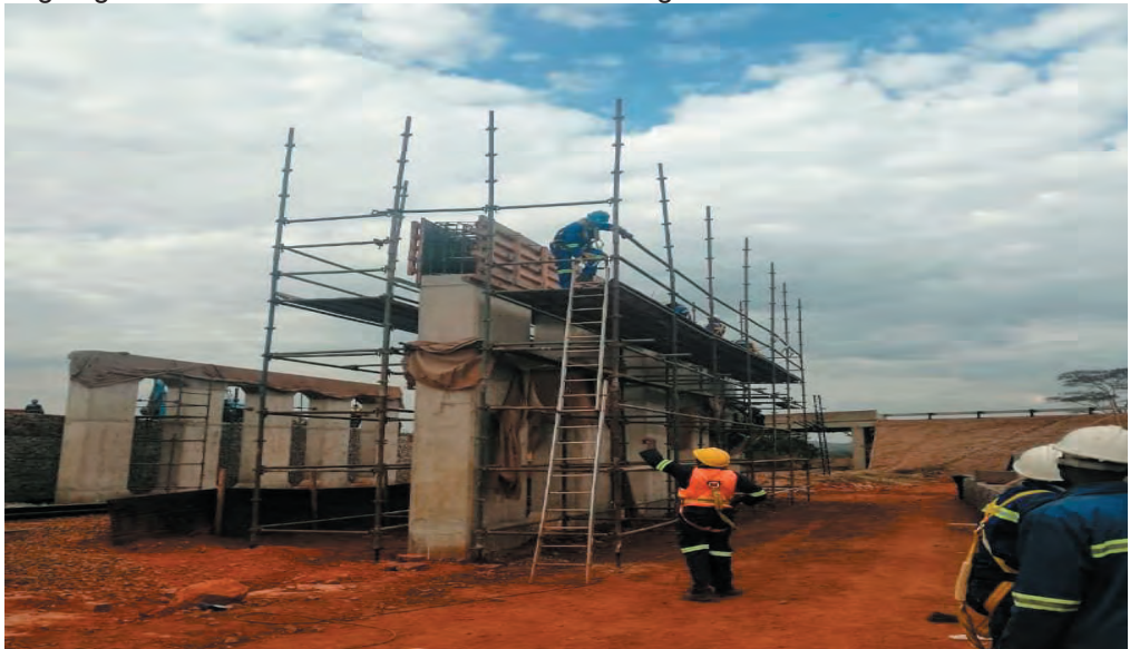
Ongoing works on the Norton Road Over Rail Bridge
