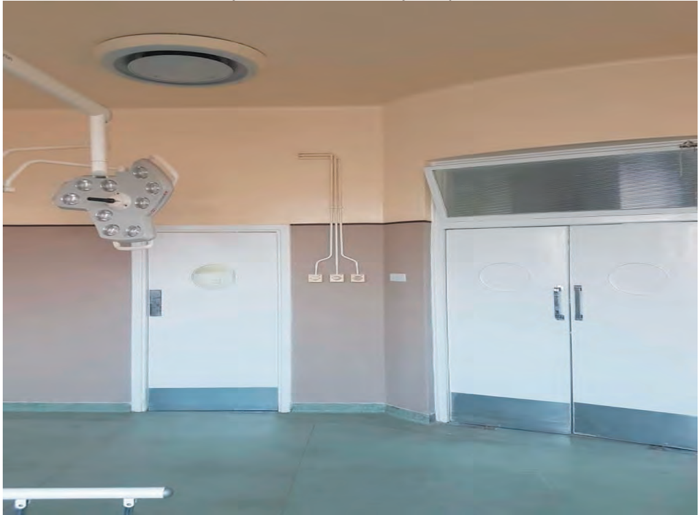
Rehabilitated theatre at Mbuya Nehanda Maternity Hospital
