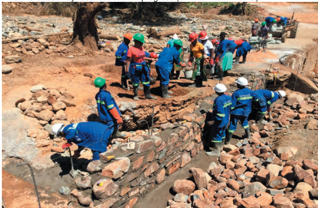
Mhakwe Causeway reconstruction in progress (Chimanimani District)
