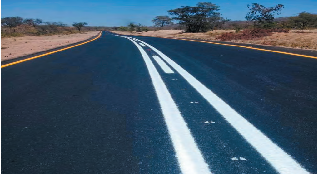
Completed section of the Bindura-Matepatepa Road
