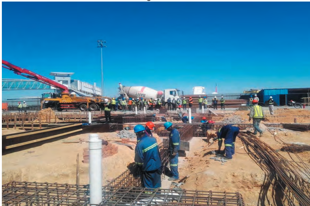
Work on foundations for terminal building extension
