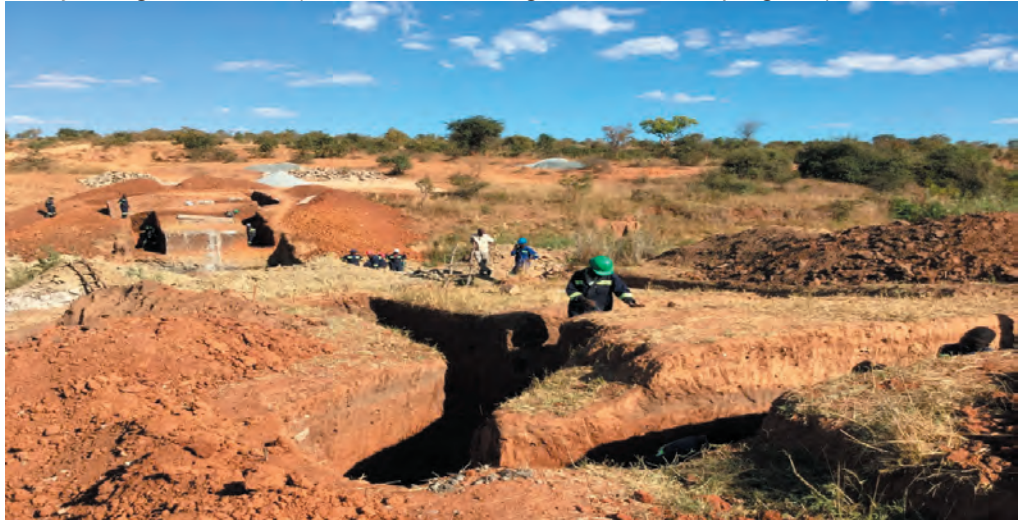
Karoyi Bridge in Guruve (excavation for Bridge abutments in progress)
